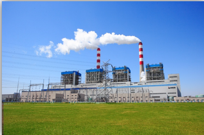
GH Cangdong Coal-fired power plant
