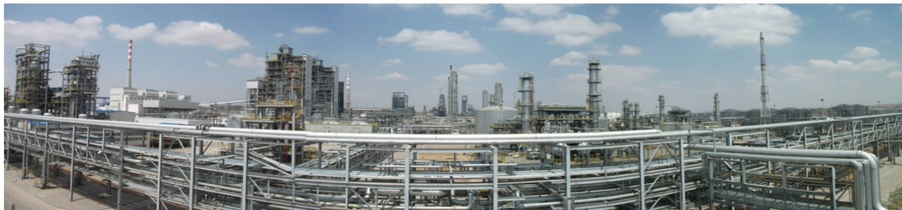
Ordos DCL demo project
