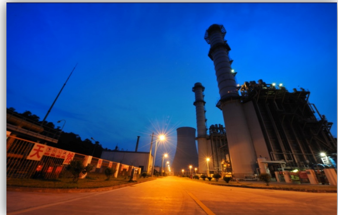
GH Yuyao gas-fired power plant
