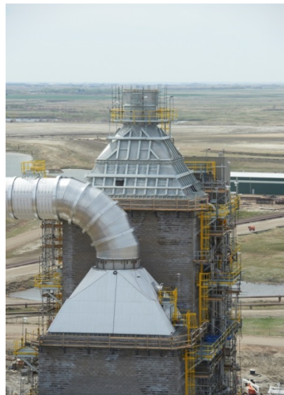
吸附塔 Absorber Towers
