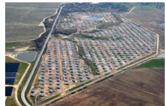
Iberinco - Cáceres Project, Spain 10MW
