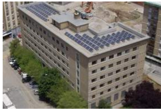
Premier Power - Pomplona, Spain 18kW
