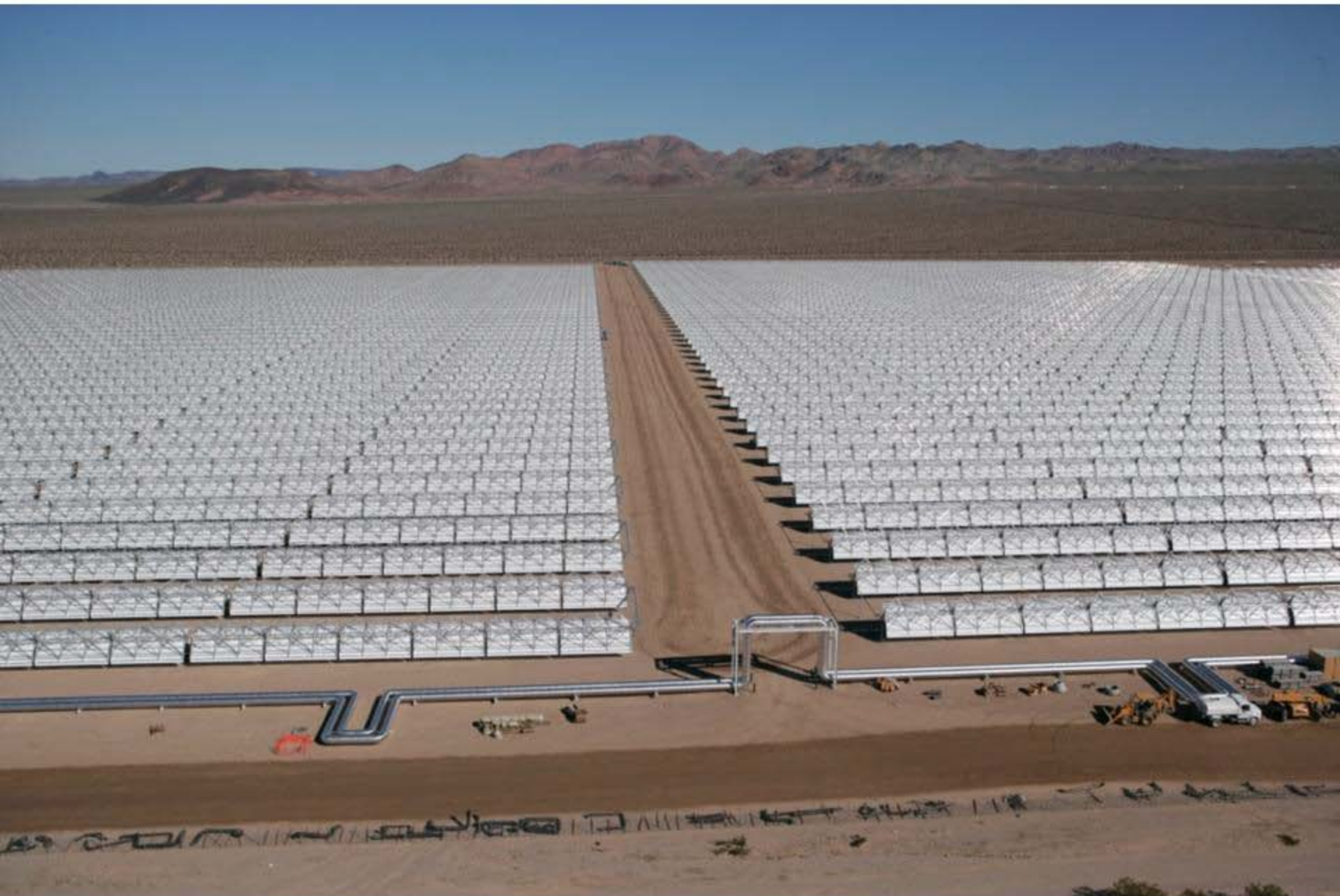
NEVADA SOLAR ONE – ACCIONA SOLAR POWER
