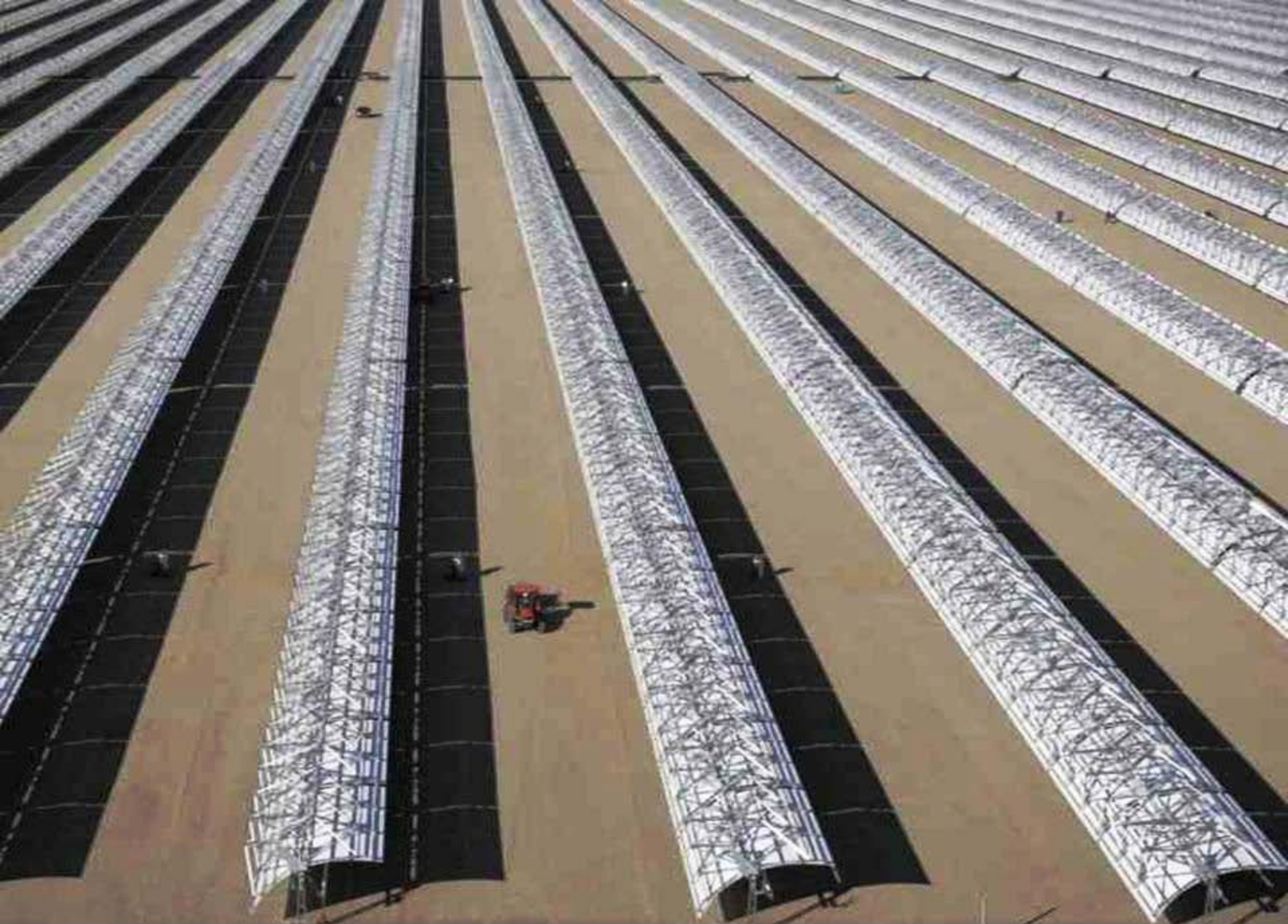
NEVADA SOLAR ONE - ACCIONA SOLAR POWER
