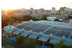
Onsite Renewable Energy
