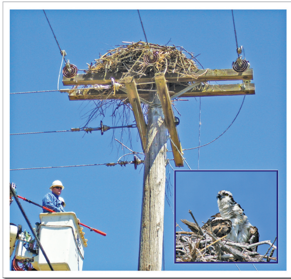
SMUD crews remove an osprey nest that presented an electrocution hazard.
