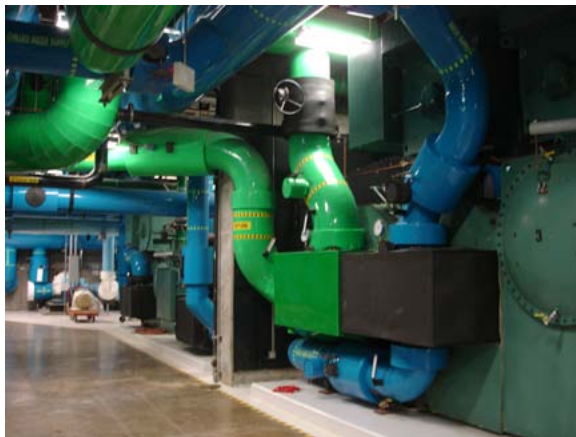
Northwind Phoenix, LLC District Cooling water circulation pipes. Blue pipes carry chilled water to client and green pipes return warm water to be chilled again.
