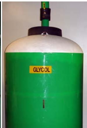
Glycol storage tank.
