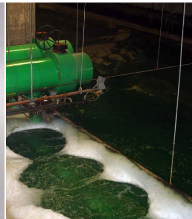
Northwind Phoenix, LLC District twenty-five foot deep glycol pool.
