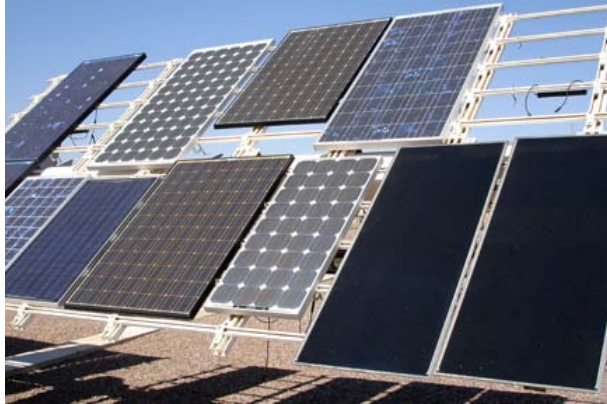
STAR Center photovoltaic cell array featuring solar cells from various manufacturers
