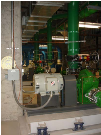
Northwind Phoenix, LLC District Cooling circulation pumps
