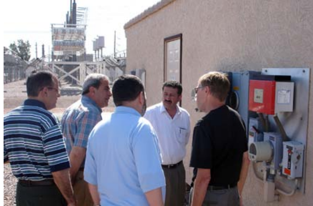
The NEPCO delegation inspects a utility controlled disconnect on a demonstration residential solar installation at the STAR Center.
