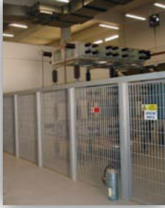
Enclosed capacitor bank at Amman South Substation
