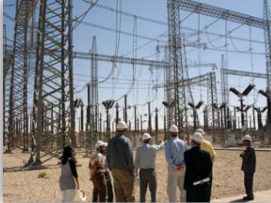
APS delegation examines the Amman South Substation yard.
