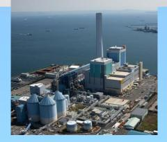
Near zero conventional emissions (NOx 20 mg/m<sup>3</sup>, sulphur oxides 6 mg/m<sup>3</sup>, particulates 1 mg/m<sup>3</sup>, at 6% O<sub>2</sub>, dry); full waste utilisation
