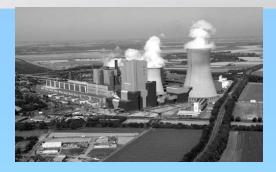
High steam conditions 27.5 MPa/580°C/600°C at turbine; initial difficulties solved using 27% Cr materials in critical areas Unique heat recovery arrangements with heat extraction to low temperatures – complex feedwater circuit
