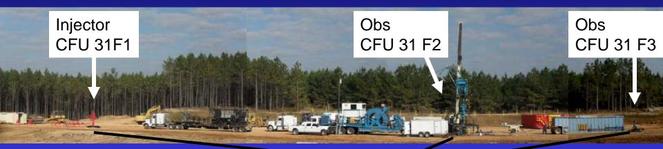
Closely spaced well array to examine flow in complex reservoir
