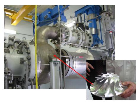
DFC-ERG®, Hybrid FuelCell, used for utility pressure reduction - more efficient pipeline operations and less air emissions
