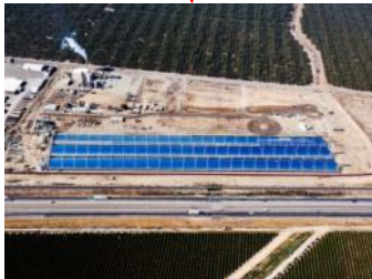
Standalone Solar & Solar Hybrid Power Plants
