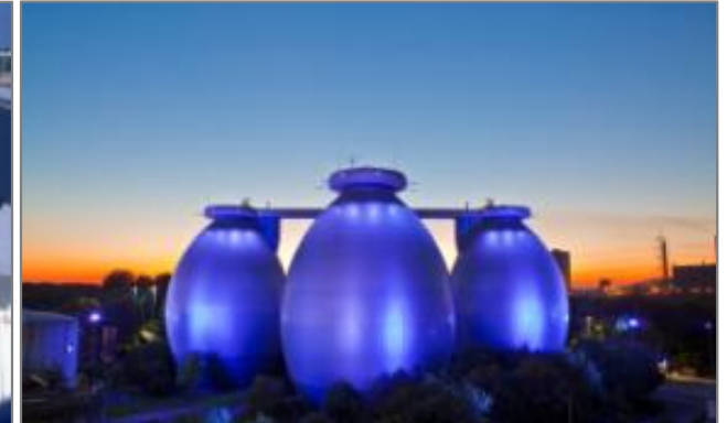
Waste water treatment plant Bottrop
