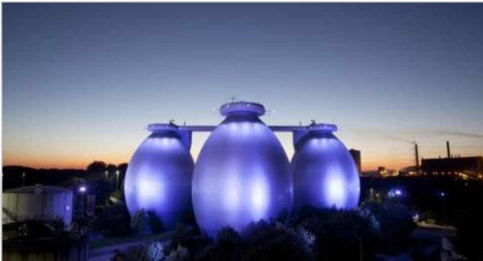
Waste water treatment plant Bottrop
