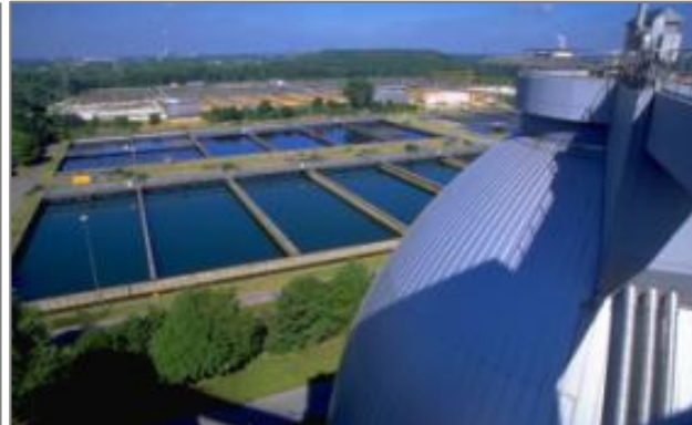
Waste water treatment plant Emscher River estuary
