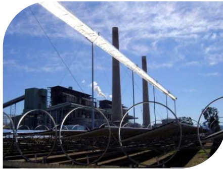
Steam Augmentation for Fossil-Fired, Geothermal and Biomass Power Plants
