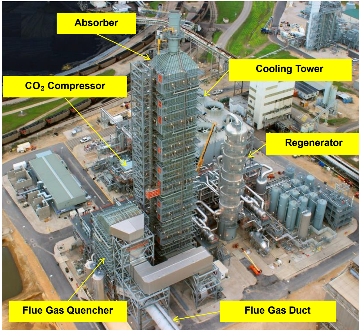
Fall 2016 View of the Site
