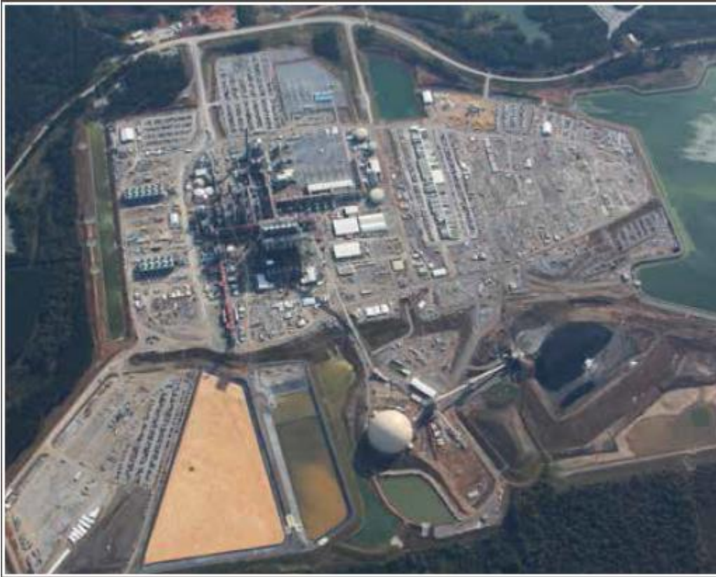
Aerial view of the facility taken in October 2013.
