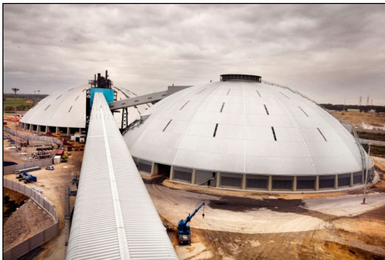
Figure 15 The coal storage domes and coal conveying systems under construction at the Torrevadalliga Nord plant (photograph courtesy of MERO)
