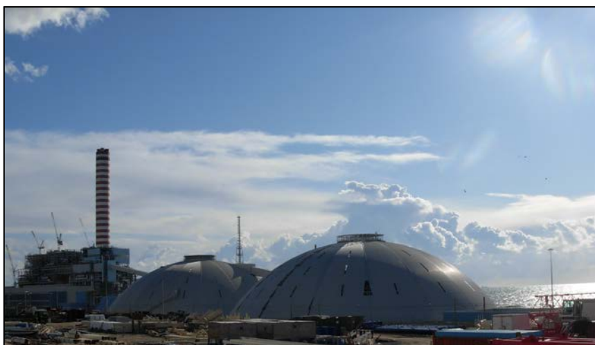
Figure 16 The completed coal storage domes at Torrevadalliga Nord (photograph courtesy of MERO)
