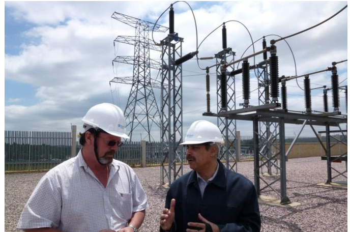
Eskom Distribution provided a tour of one of its newest substations in the suburbs of Johannesburg, the Beyers Substation featuring 11kV switchgear, built to handle urban development that coincided with the 2010 FIFA World Cup.
