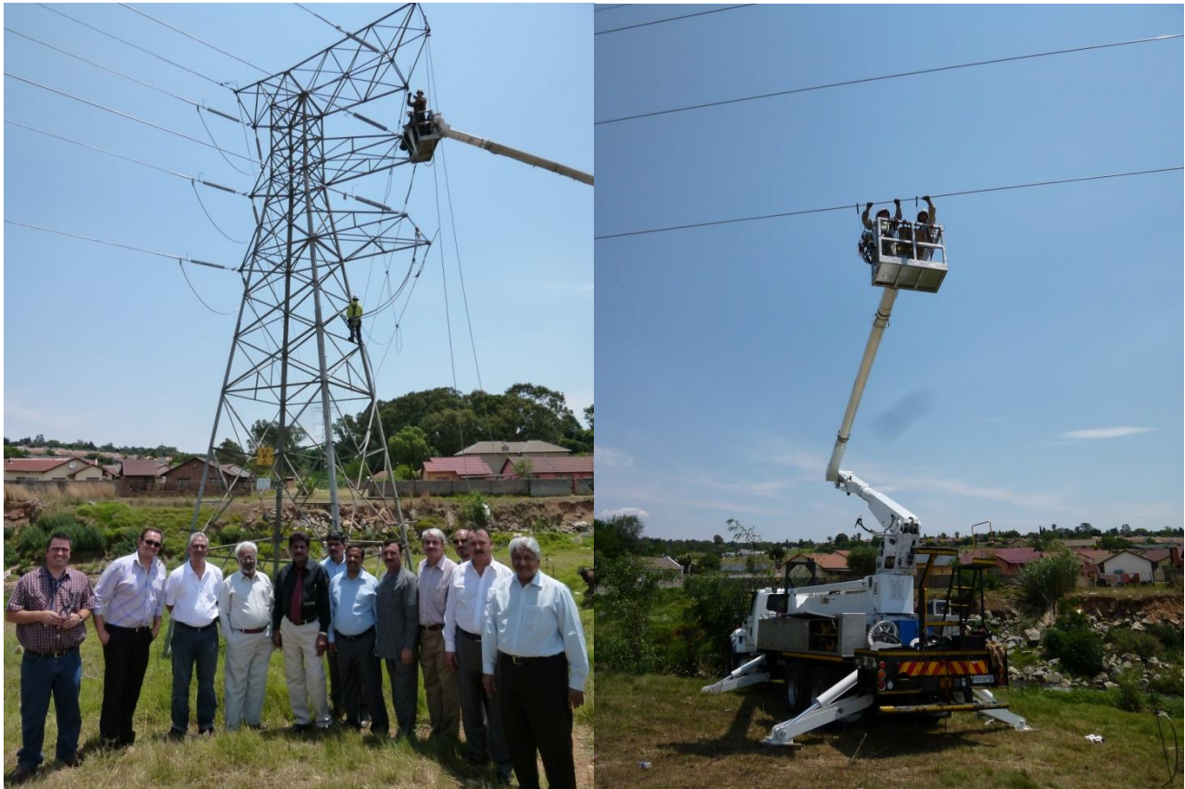
The delegation witnessed live-line transmission repair and maintenance work performed by Quanta Services for Johannesburg City Power. The techniques employed here improved electricity delivery in South Africa during the 2010 World Cup, and could be utilized in Pakistan to minimize outages during line work.
