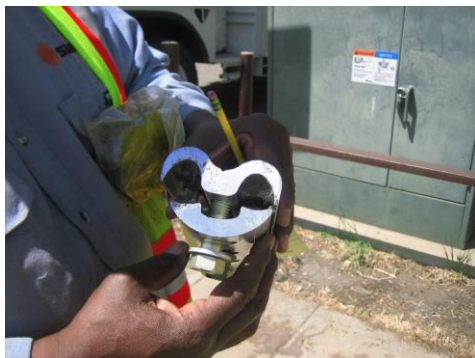
Parallel Groove connector used by SMUD.
